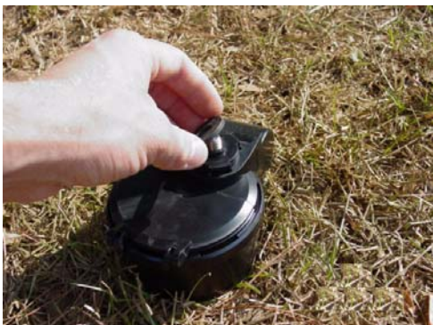
Figure 15 Placing Washer on MIU
