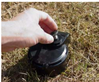
Figure 9 Placing Washer on MIU
