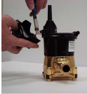
Figure 7 Using Scotchlok to Splice Wires
