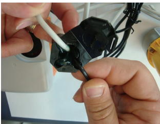
Figure 15 Wires in Slots
