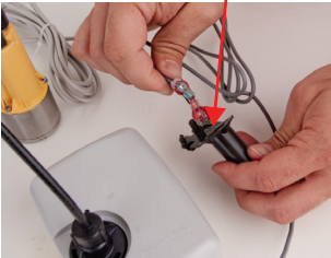
Figure 13 Splice Tube
