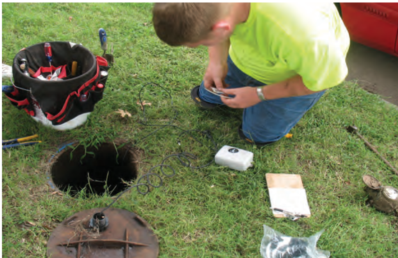
Installation of an R450 in a pit.
